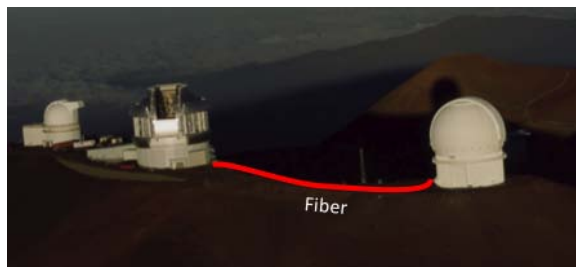
Figure 9-4: A first in astronomy, two major independent observatories on Mauna Kea will be joined by a fiber, feeding a high resolution optical spectrometer at CFHT with photons collected at Gemini-N.
